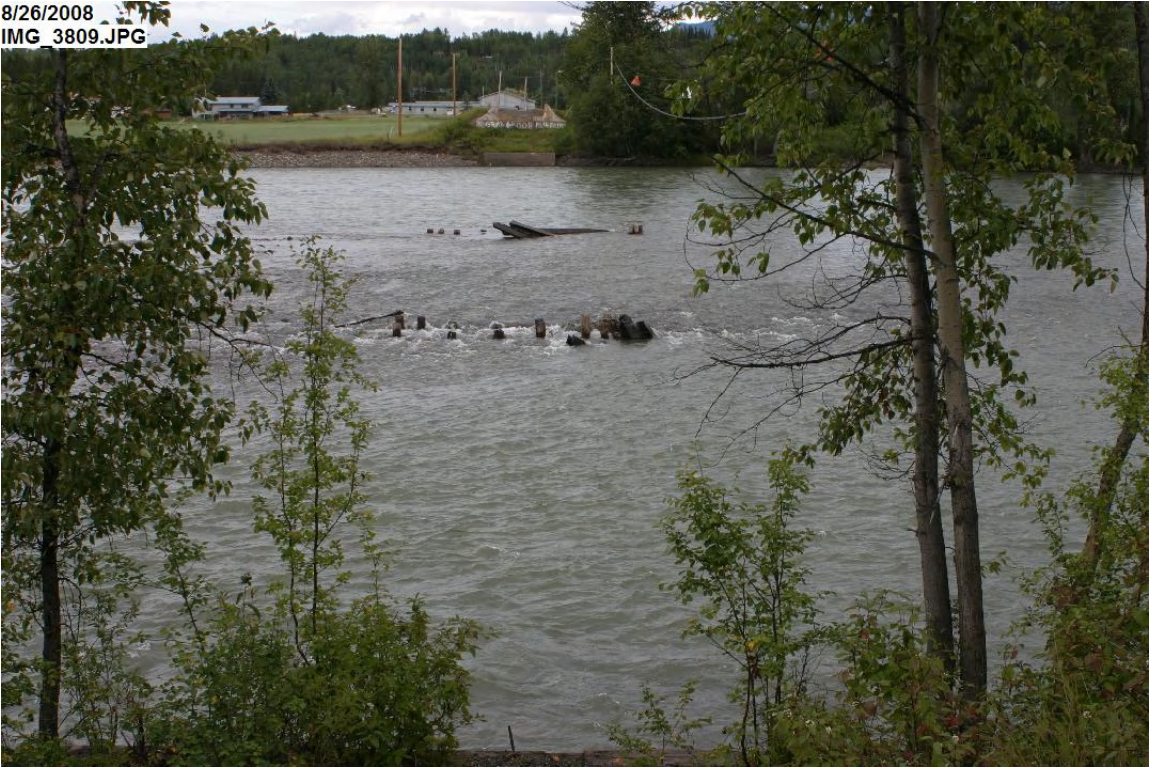
Bulkley crossing from south side – note old bridge piers
