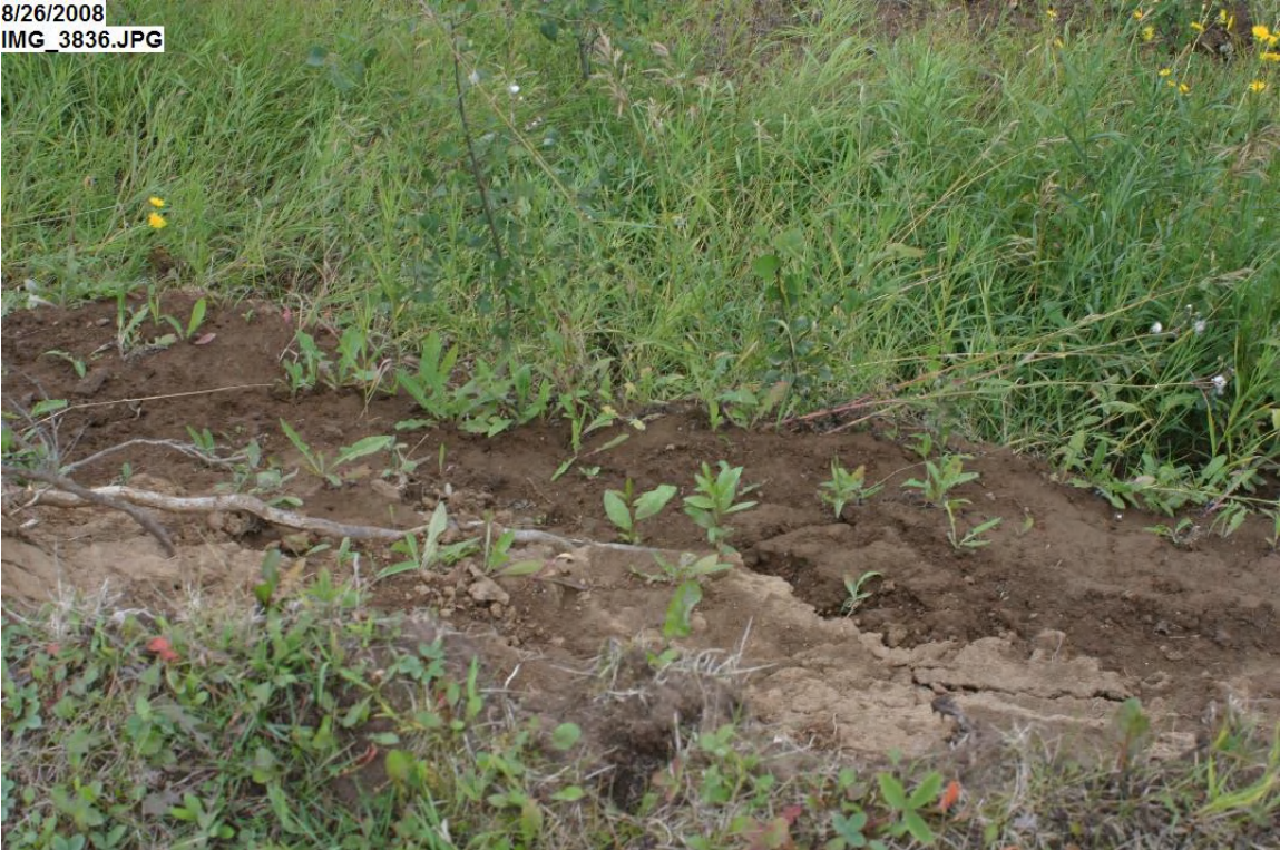
Riverside park entrance – steep and unstable bank
