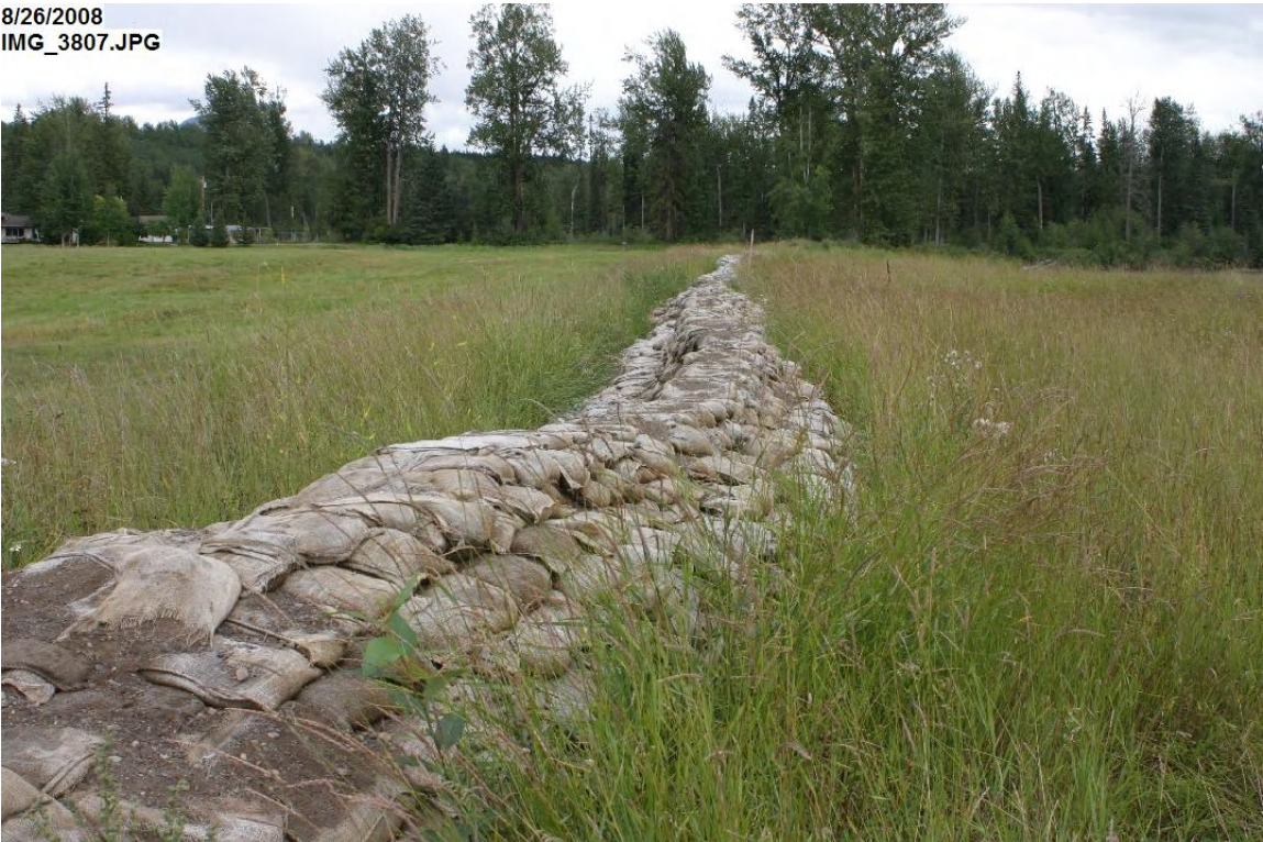
Sandbag dike at the end of Kidd Road
