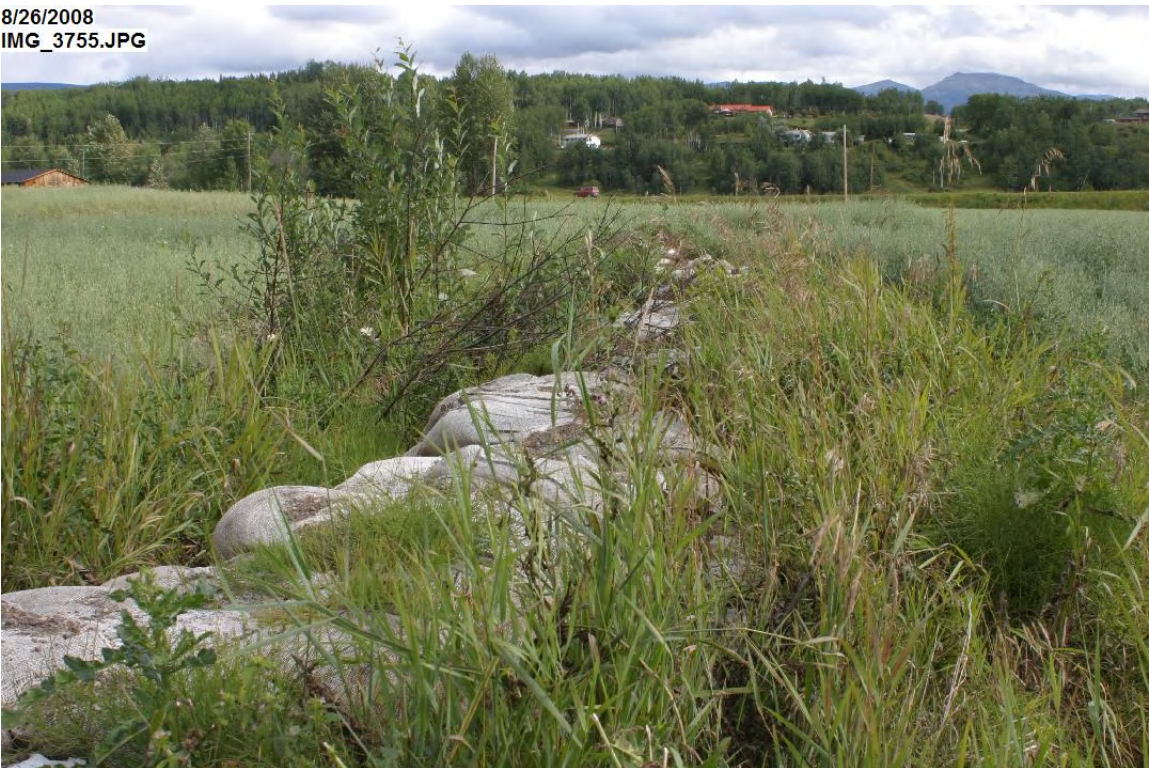
Sandbag dike looking east
