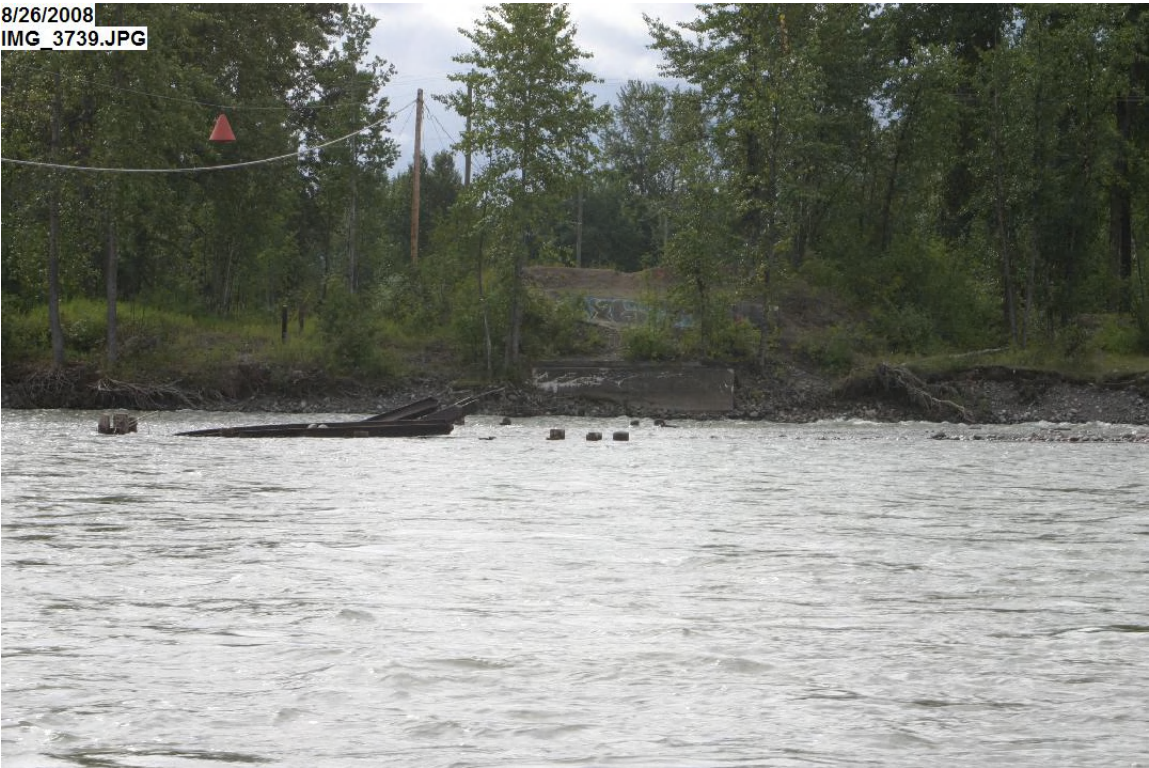
View of left (south) bank showing old abandoned bridge piers
