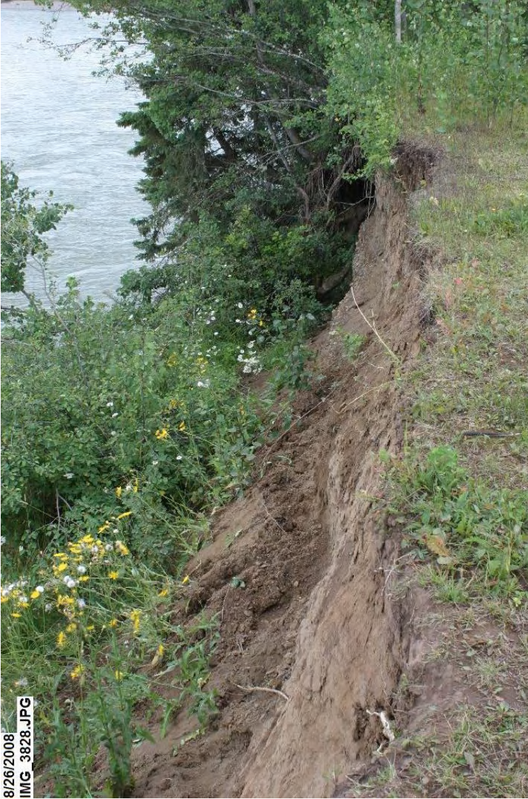
Slope failure east of Riverside Park
