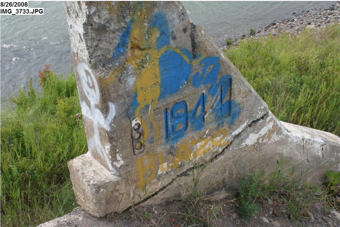
Old bridge wingwall
