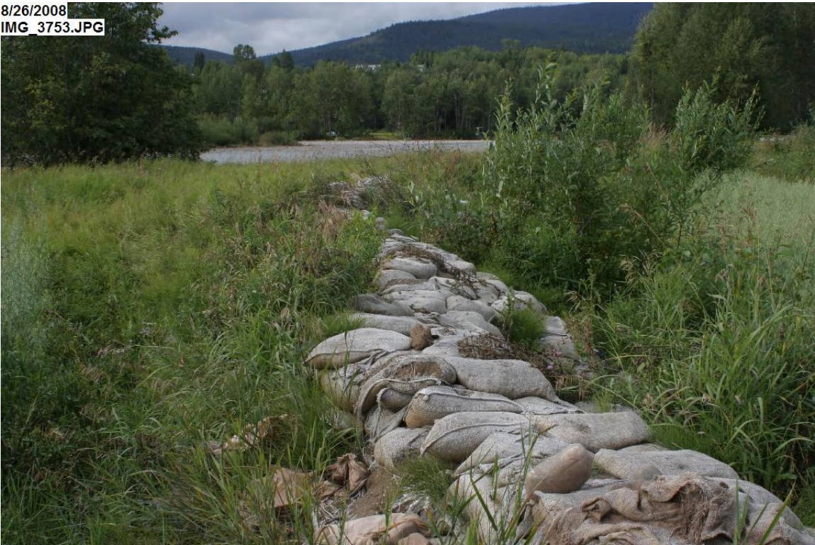
Start of sandbag dike
