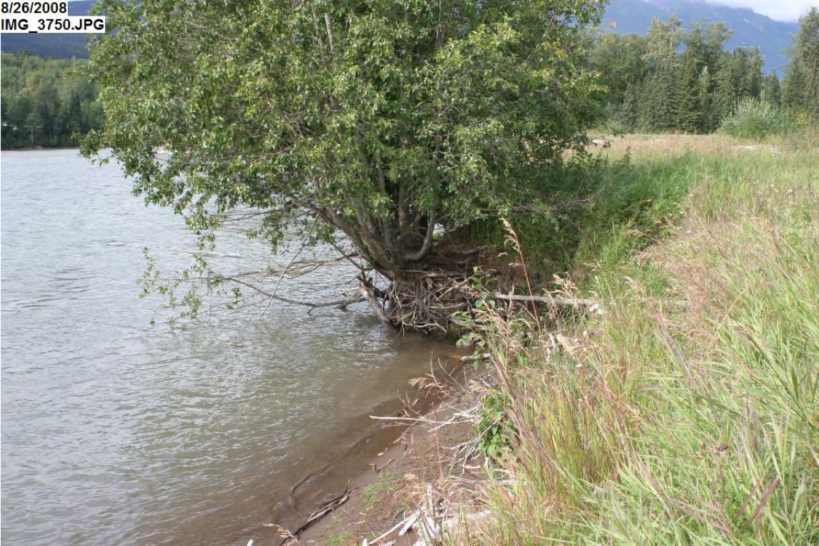
Beginning of undercutting of bank – bank material is silty sand
