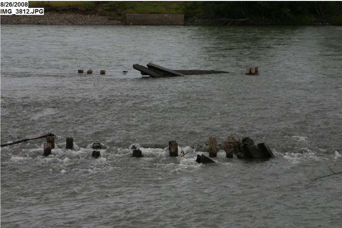
Lateral flow was noticed coming over the bridge piers and shallow gravel bar
