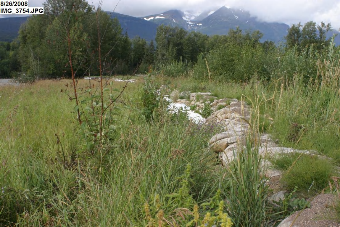
Sandbag dike looking west
