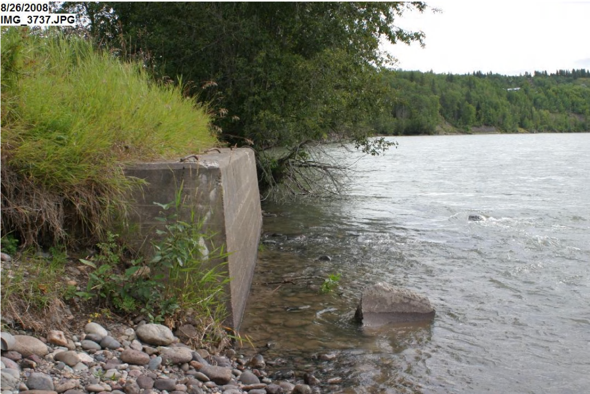
Bridge abutment at old crossing
