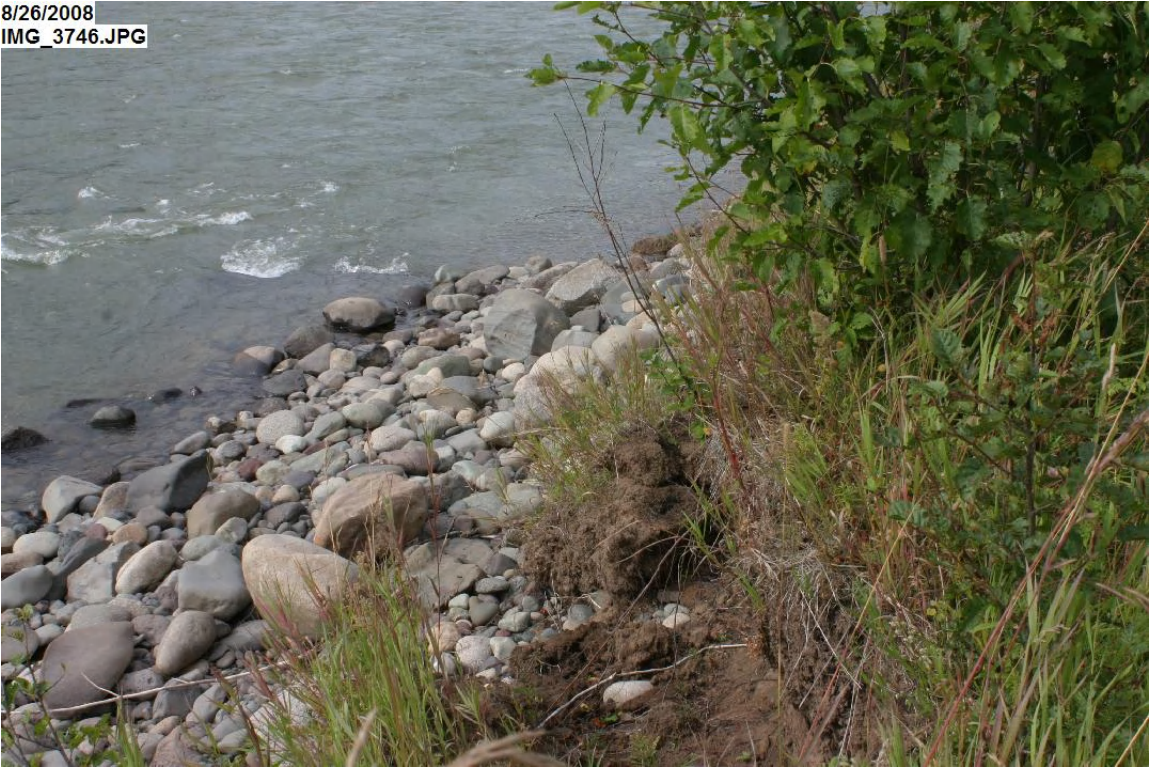
Substantial increase in bank rock size in this location
