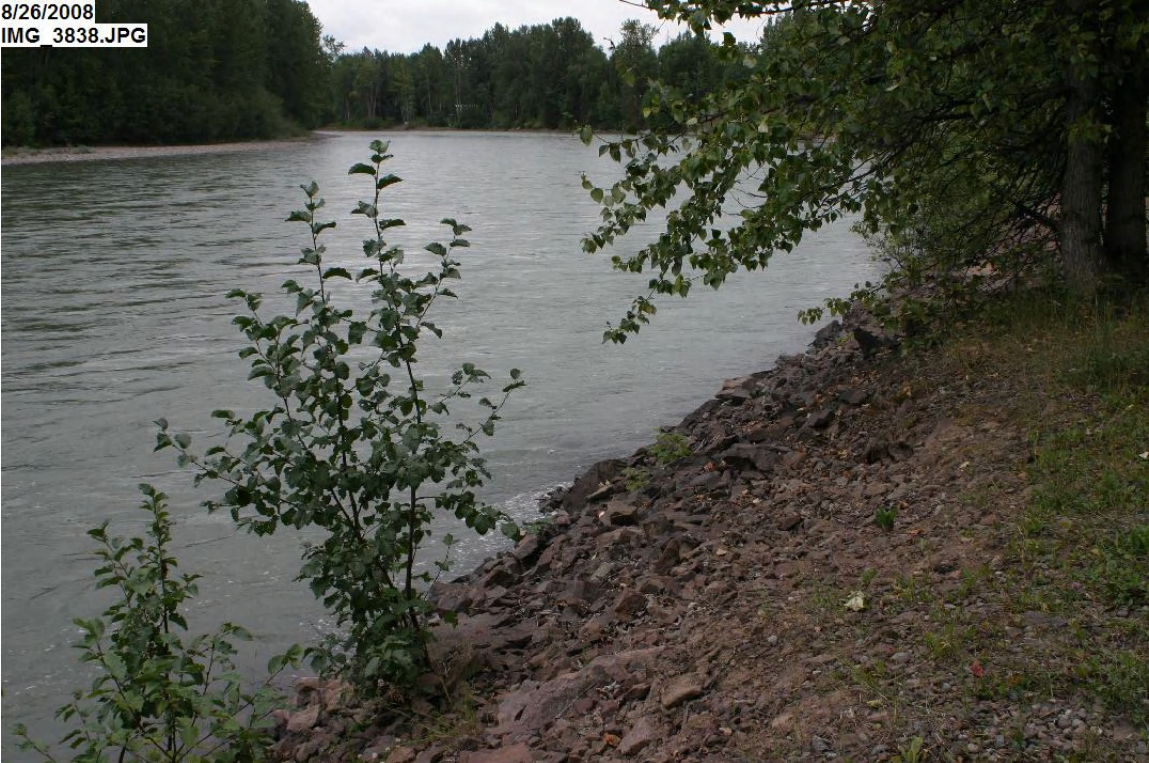
Riprap at Riverside Park
