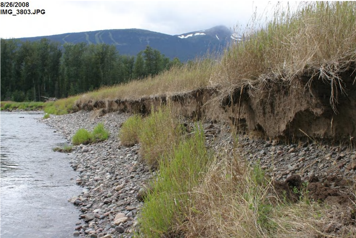
Bank undercutting at end of Kidd Road
