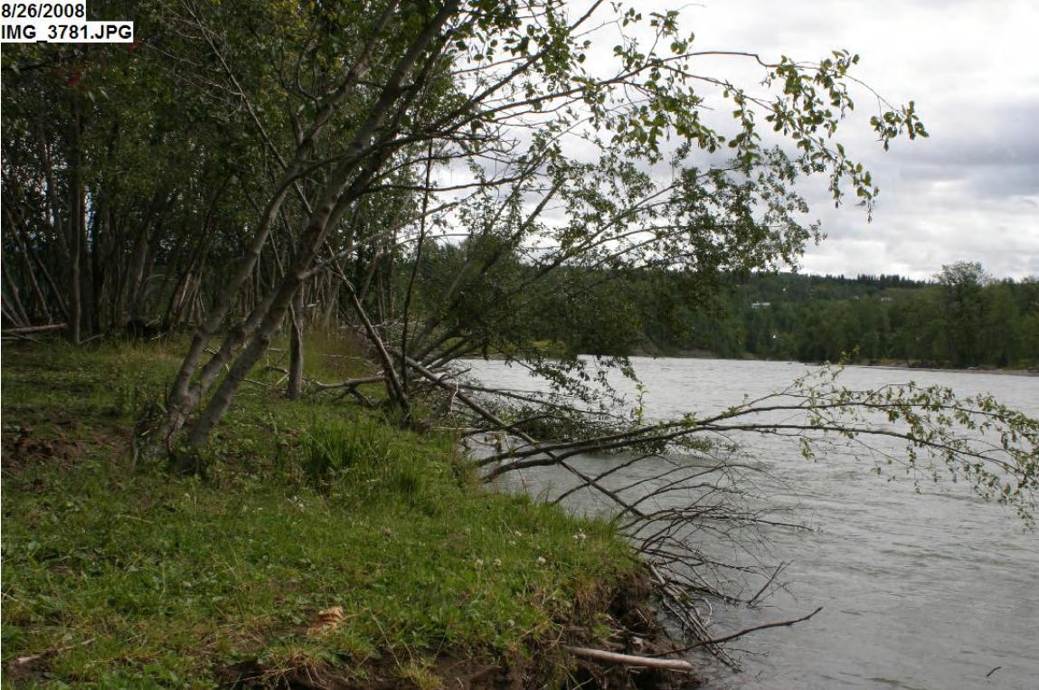
Leaning trees indicate continued erosion and bank failure
