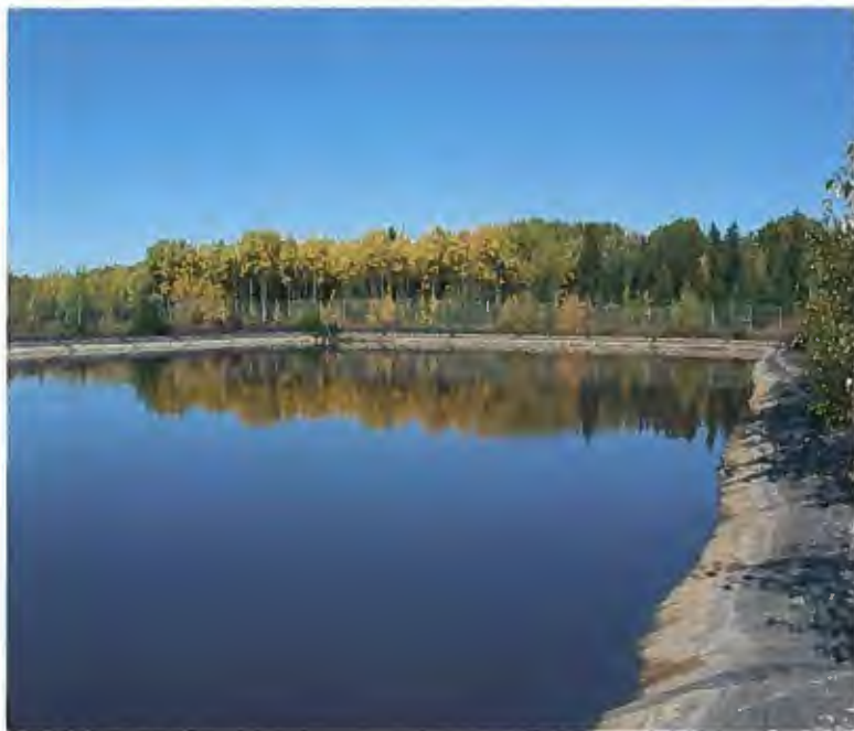
(Knockholt Septage/Leachate Lagoon)
