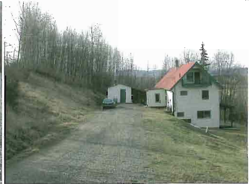
Photo 7: View southwest at driveway and house at 1037. Development created by cutting and filling on old river valley slope.
