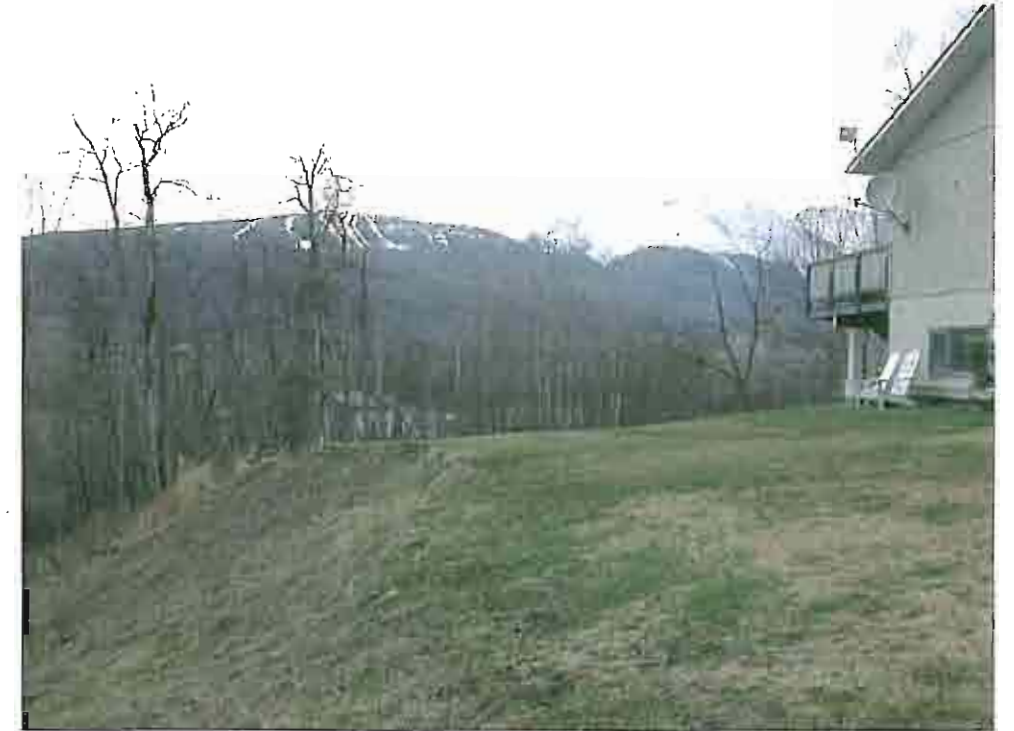
Photo 29: Looking west at main scarp of landslide adjacent to 355. Scarp area has been regraded by landowner. Septic line crosses this slope.
