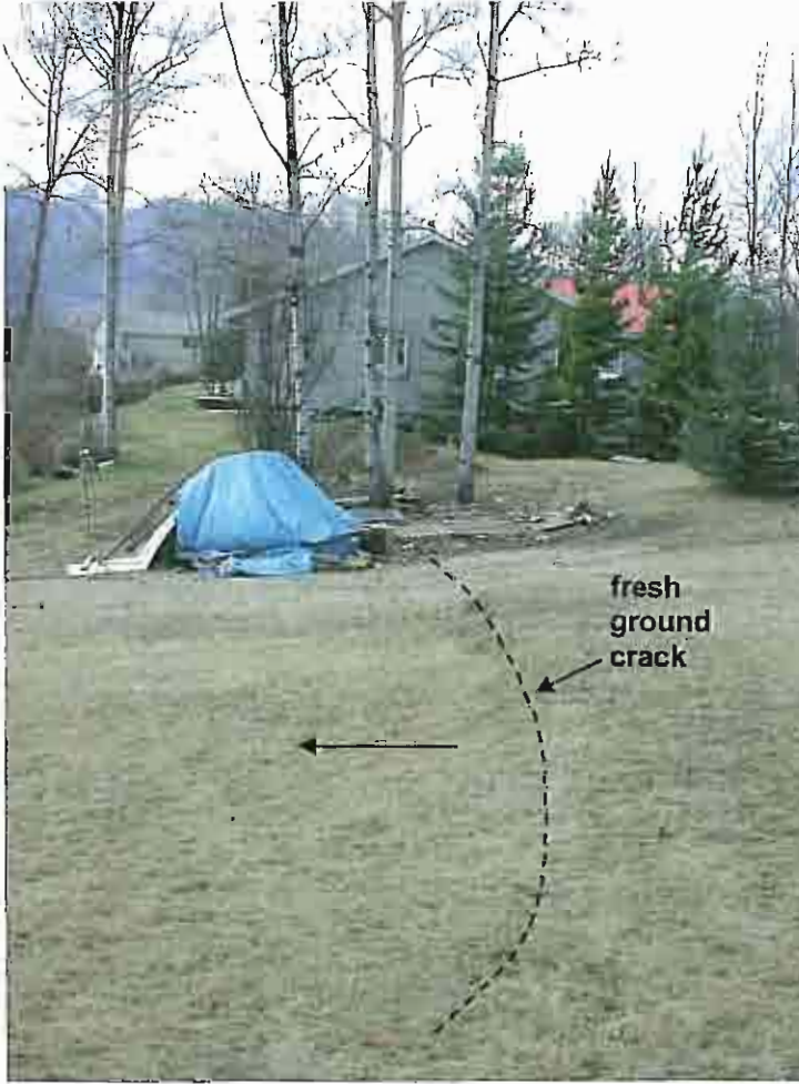
Photo 25: Looking north west along fresh ground cracking between 195 and 265.
