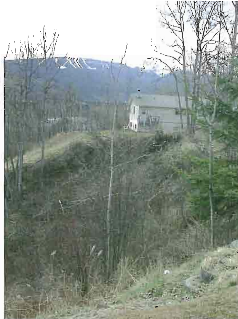
Photo 28: Looking west along main scarp of landslide between 265 and 355.
