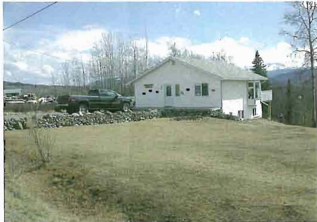
Photo 14: View southwest at 195 Lower Viewmount Road, house located at crest of river valley slope.
