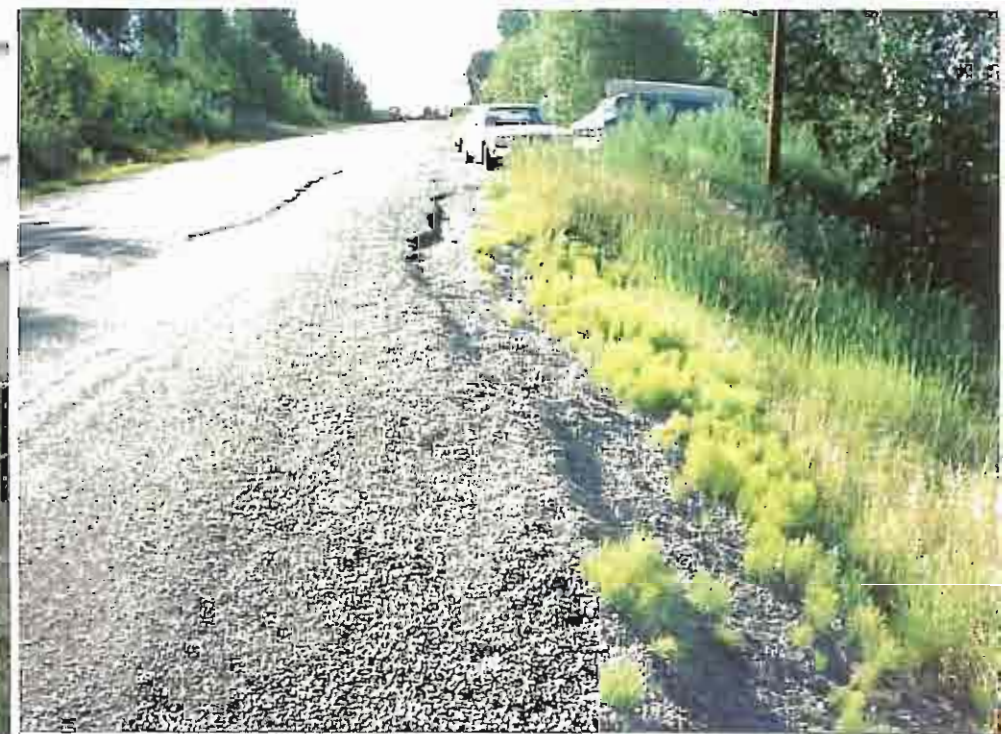
Photo 10: MoT file photo (ca. 1989), looking south at fill failure on Lower Viewmount Road near driveway access for 1037.
