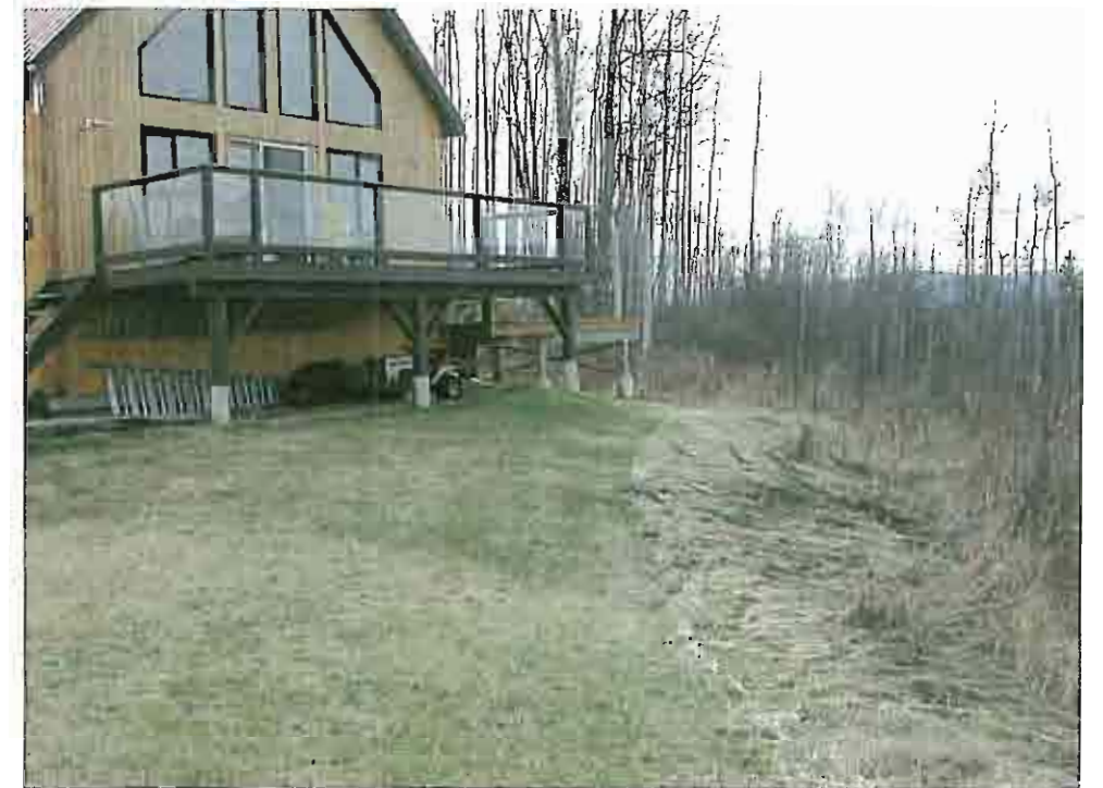
Photo 31: View east at house 485 located at the crest of the valley slope, possible main scarp location but less distinct. Septic and water lines cross this slope, septic lagoon located on slope to right of photo.
