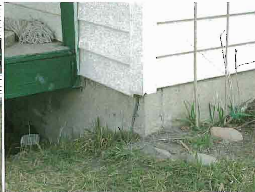
Photo 9: Small crack in south west corner of concrete foundation of 1037.
