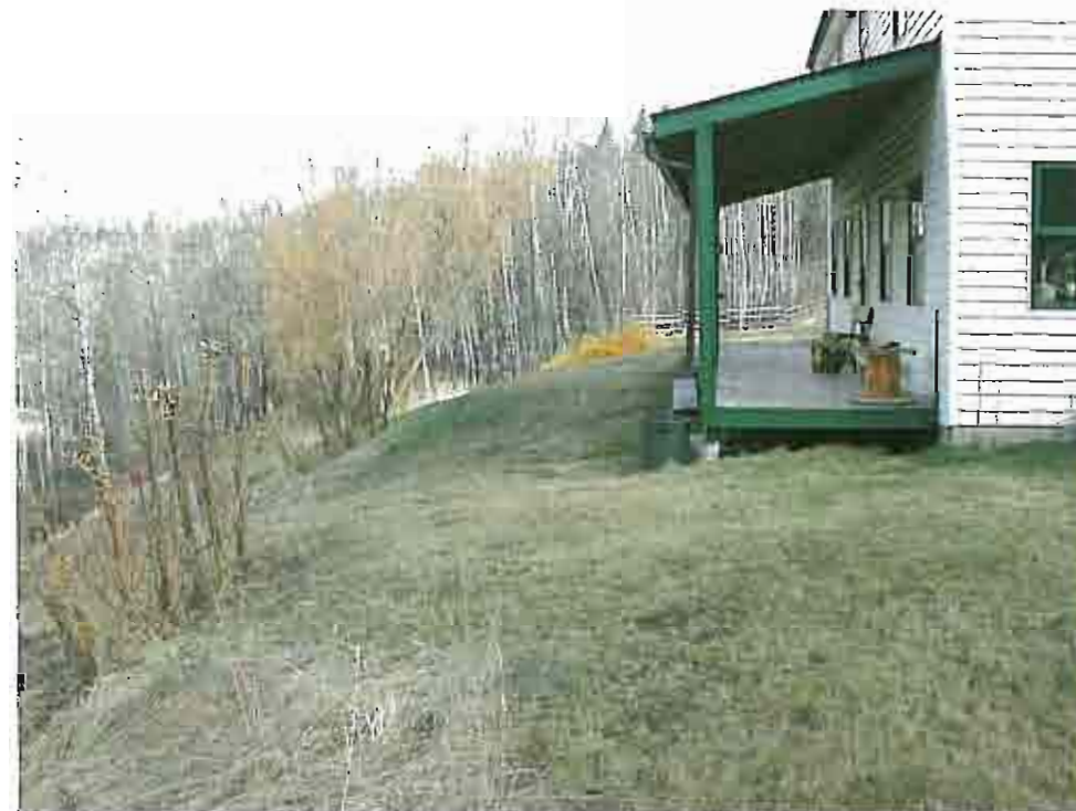
Photo 8: View north at fill on west side of 1037. Possible slow fill settlement and/or sliding downslope of house.
