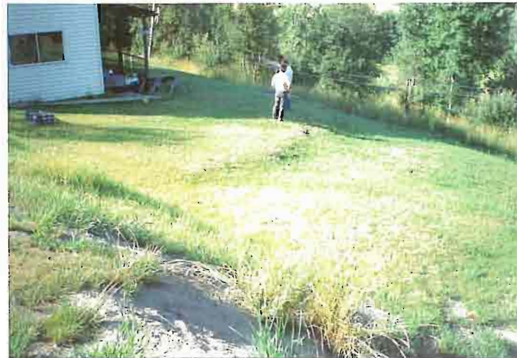
Photo 13: MoT photo (ca. 1989), looking south west at ground movements in fill north and west of 1037. Note, present day septic disposal and possibly water service lines may cross this area.
