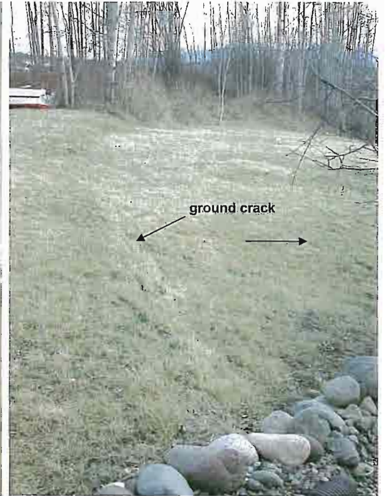
Photo 22: View south along fresh ground cracking (likely new main scarp of landslide) from south east side of 195. Note, the house septic disposal line crosses this area.
