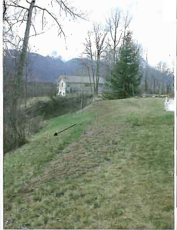
Photo 26: Looking north west at main scarp of landslide, just behind (downslope) of 265. Evidence of recent ground disturbance or movement.
