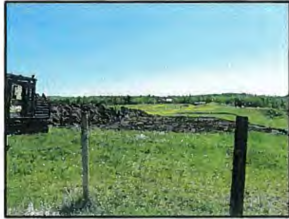
Cleared area for riding arena
