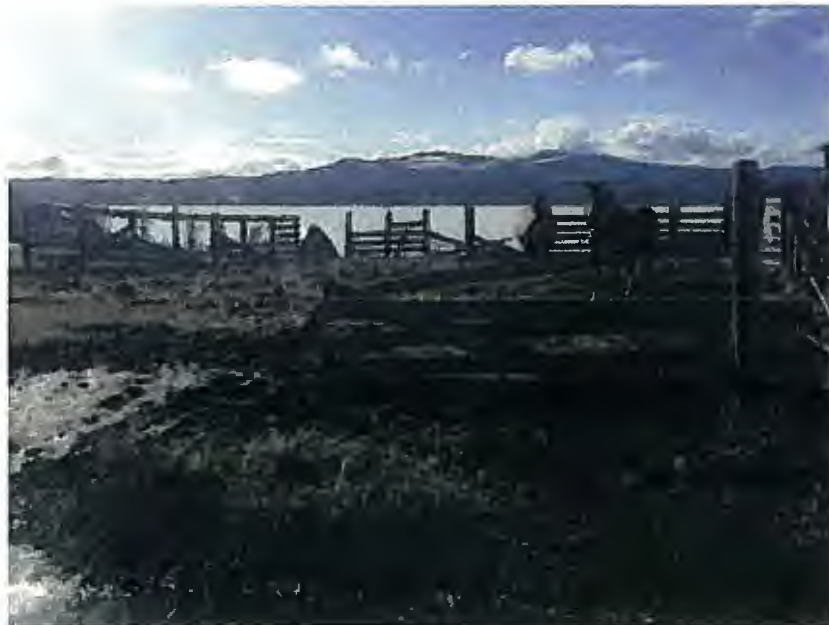
Phot 3 - Building 2 and Surrounding Fences
