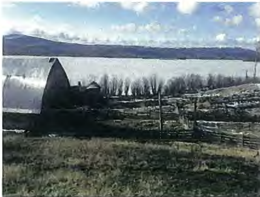
Photo 15 – Old Barn, Collapsed Building
