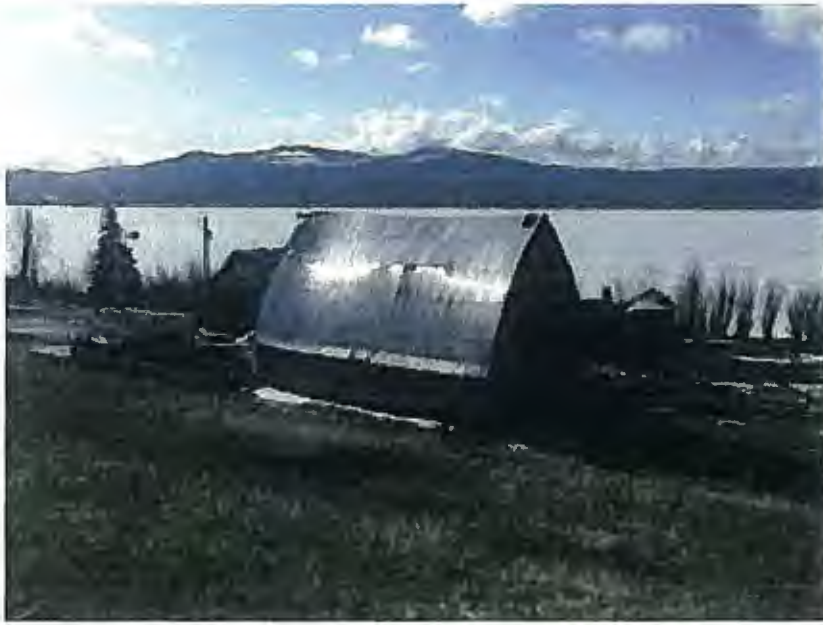
Photo 16 – Old Barn, Collapsed Building, House in Background
