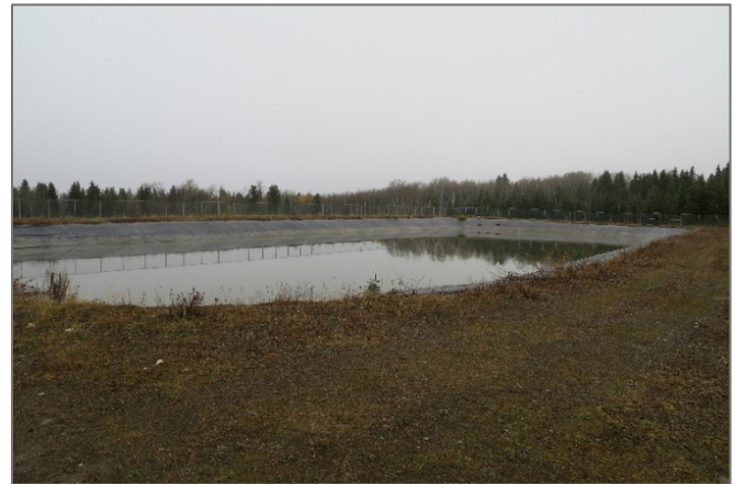
Photo 2-9: Knockholt Landfill Leachate Pond (photo by Tetra Tech 2017)
