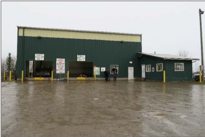
Photo 2-4: Vanderhoof Transfer Station Building (photo by Tetra Tech 2017)
