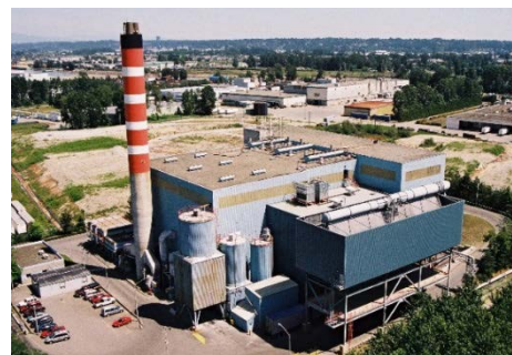
Photo 4: Burnaby WTE Facility.
