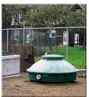
An appropriate and effective on-site sewage disposal system is very important for waterfront properties. Domestic sewage is an important contributor of phosphorous to lakes and watercourses because primary and secondary treatment removes only about 20 to 30% of the element from sewage.
