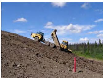
Final closure works at the old Burns Lake Landfill were completed including the establishment of suitable grading, placement and compaction of low permeability soils on previously landfilled areas, and grass seeding. Work to update the Environmental Monitoring Plan for the site was also undertaken in 2012, which included the establishment of three new groundwater monitoring wells at the site.
