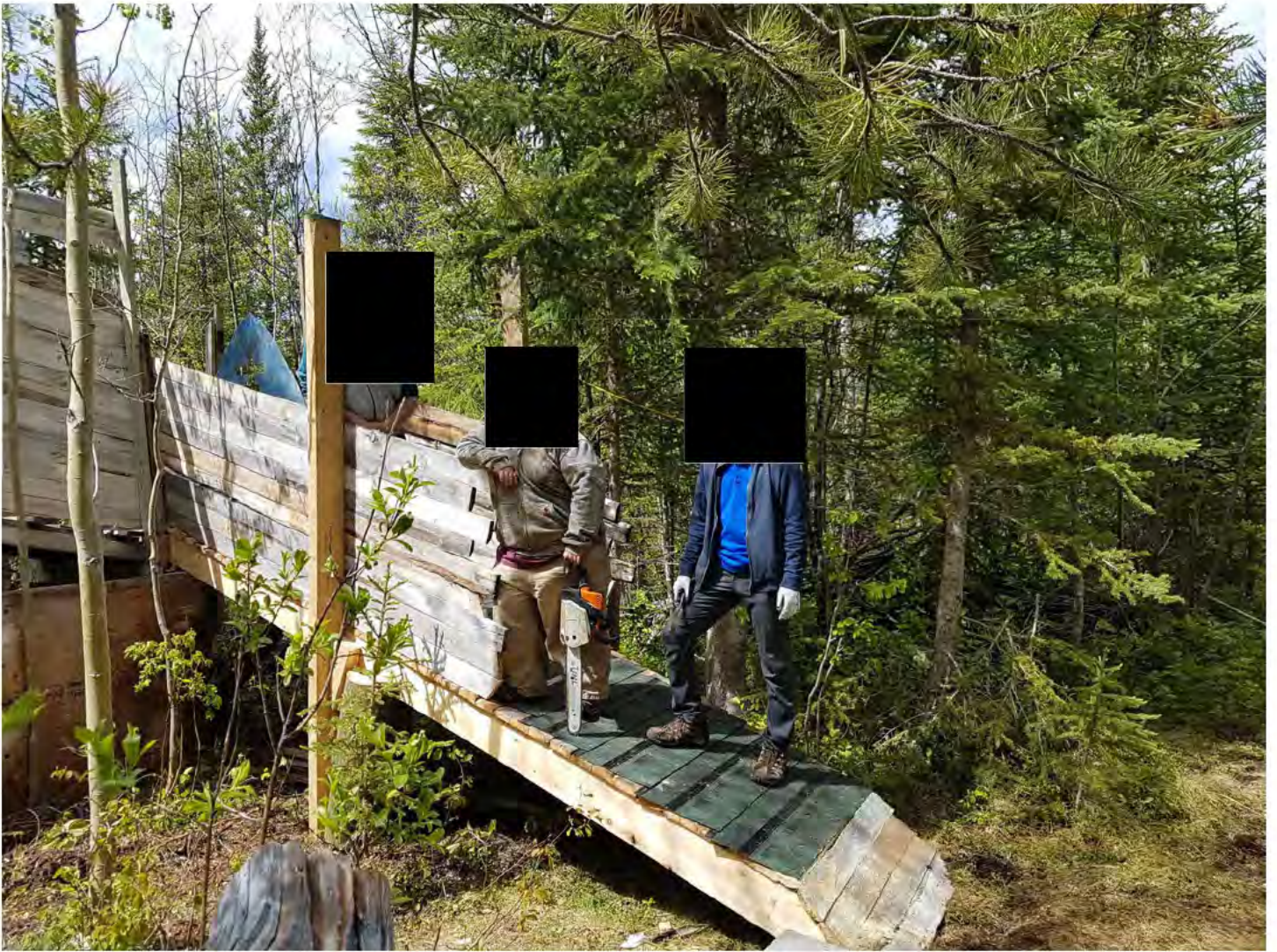
Installation of a longer replacement ramp on the north east side, summer 2020
