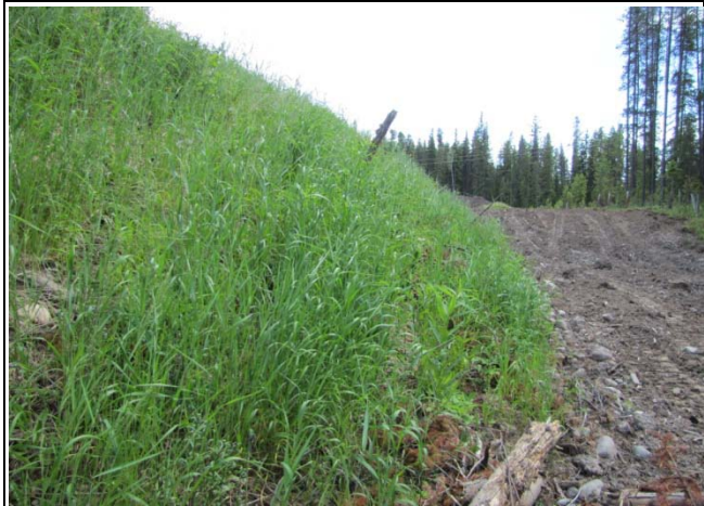
Vegetative growth on the west soil/till berm
