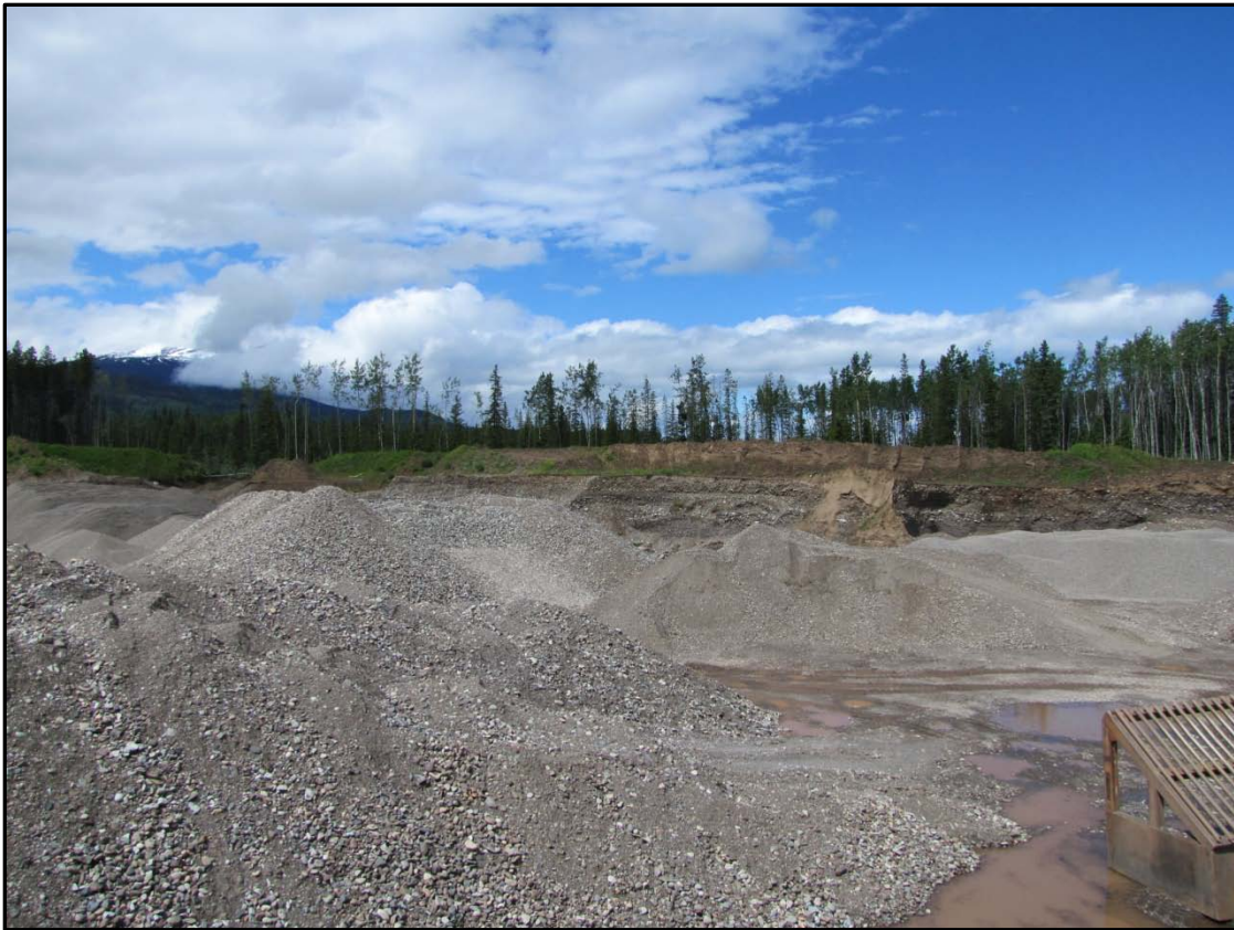
Looking north-west across part of the existing pit operations
