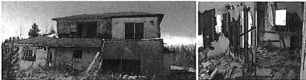
The estimated cost for the RDBN to hire a contractor to demolish and remove the structure is \$7,700 (\$3000 tipping fee, \$2250 excavator, \$2400 two dump trucks). This estimate is based on 12 hrs of work.
