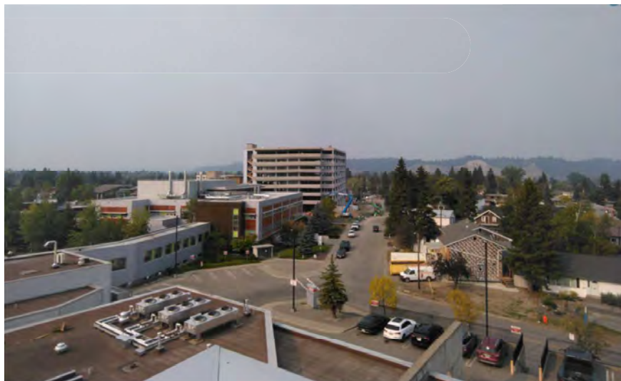
Parkade Construction Site
