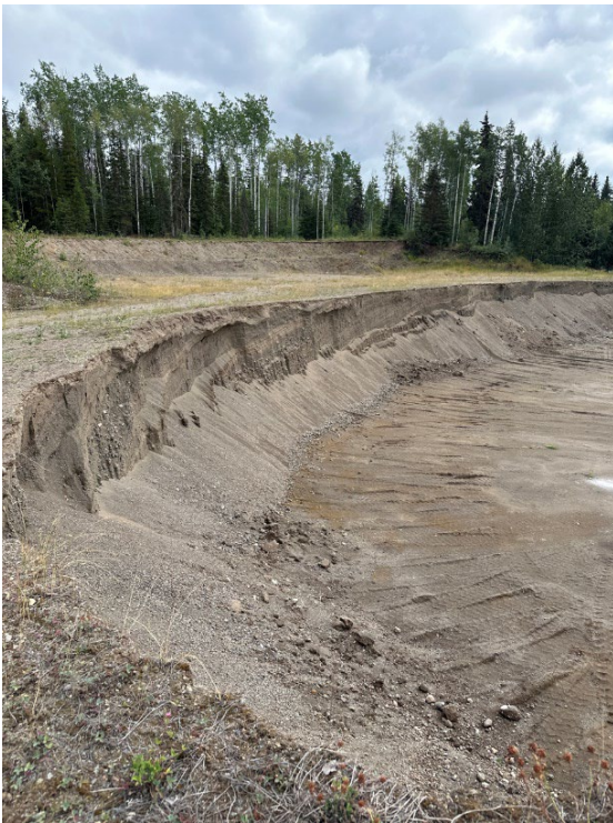
Plate 2.2-3. Pit wall showing glaciofluvial sediment used for gravel excavation.
