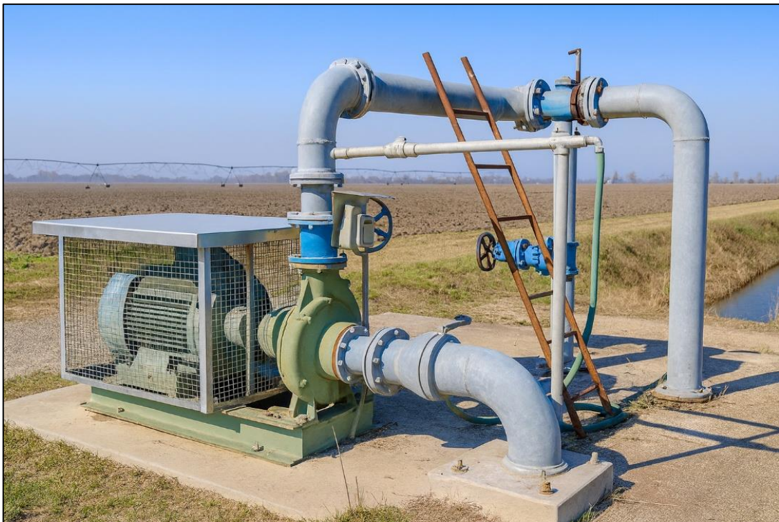
Figure 10. Example of pump and connection to main water pipeline that would be located at the farm parcel level.
