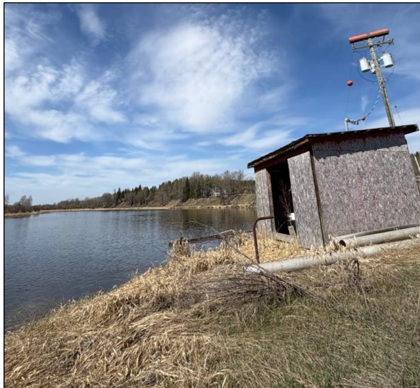
Figure 11. Existing pumphouse on the Nechako River used to convey water to agricultural properties at a higher elevation.
