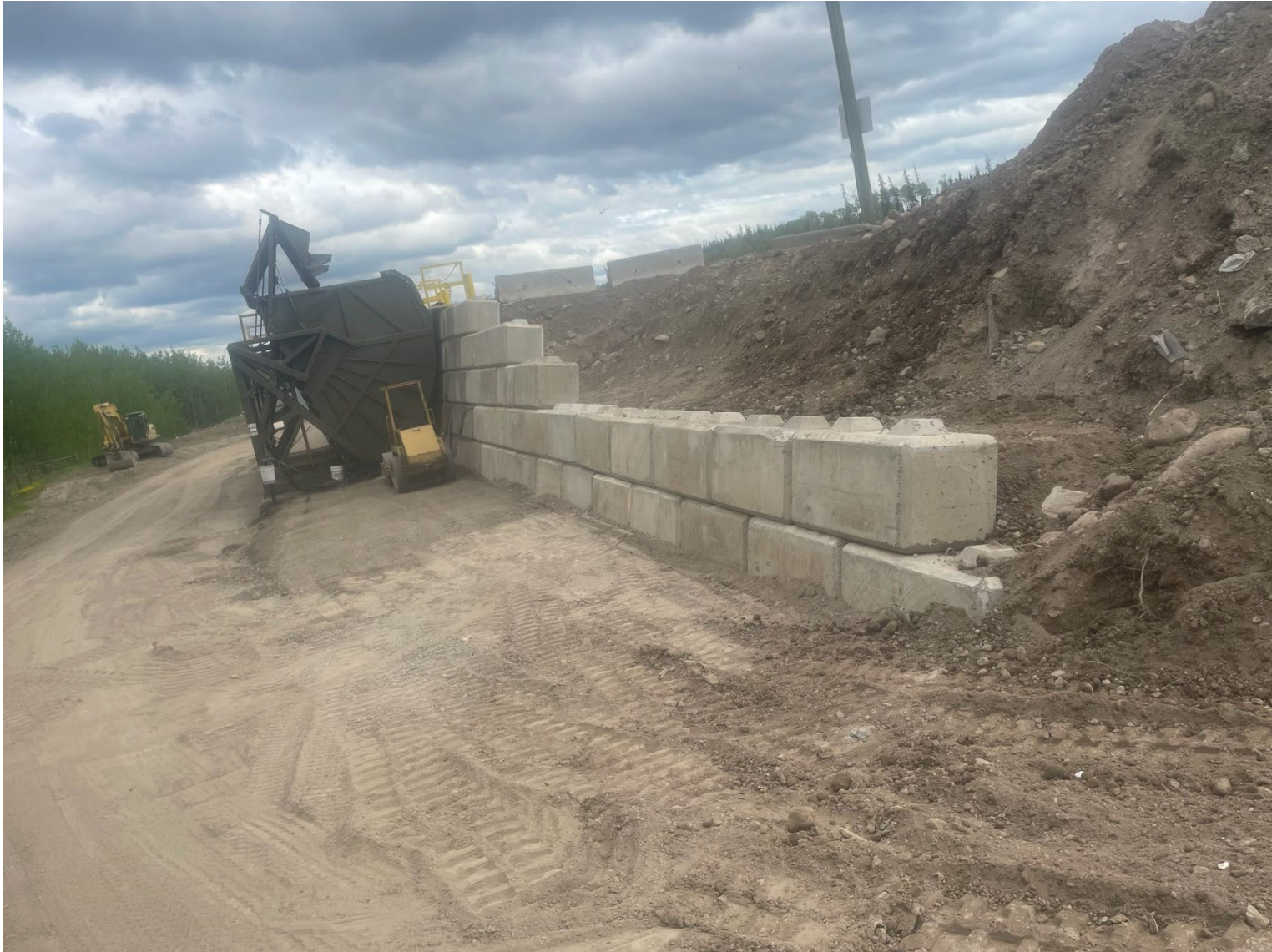
Photo 1. Existing infrastructure facing west
