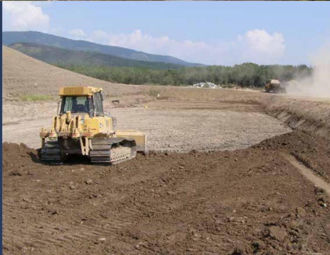
**The project was completed in 2022** with a combination of contractors and RDBN Landfill staff. The expansion covers about 70,000 square meters and will hold approximately 250,000 tonnes of solid waste.
