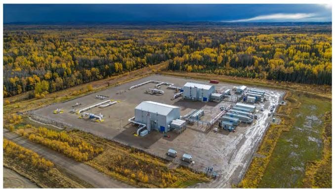
Figure 1: TC Energy Operating Compressor Station (Note: This figure depicts a 2 unit facility, and the Proposed Clear Creek Compressor Station may have up to 3 units)
