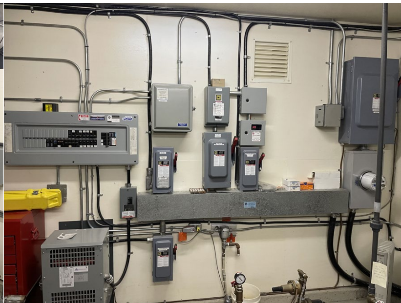
Figure 5 - Hypochlorite Dosing tank/pumps (internal supply Piping).....Figure 6 -- Breaker Panel and Cycle Stop Switches
