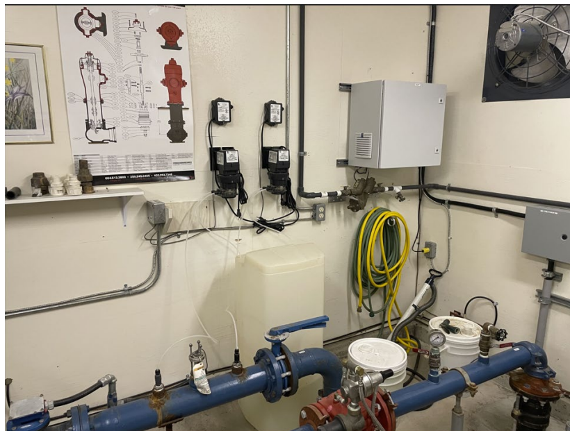
Figure 5 - Hypochlorite Dosing tank/pumps (internal supply Piping).....Figure 6 -- Breaker Panel and Cycle Stop Switches
