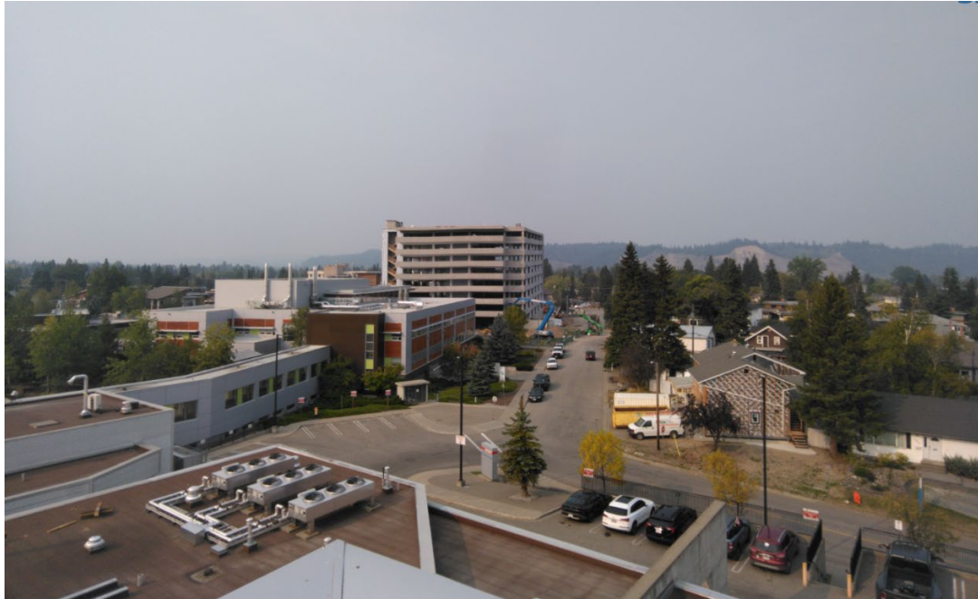
Parkade Construction Site
