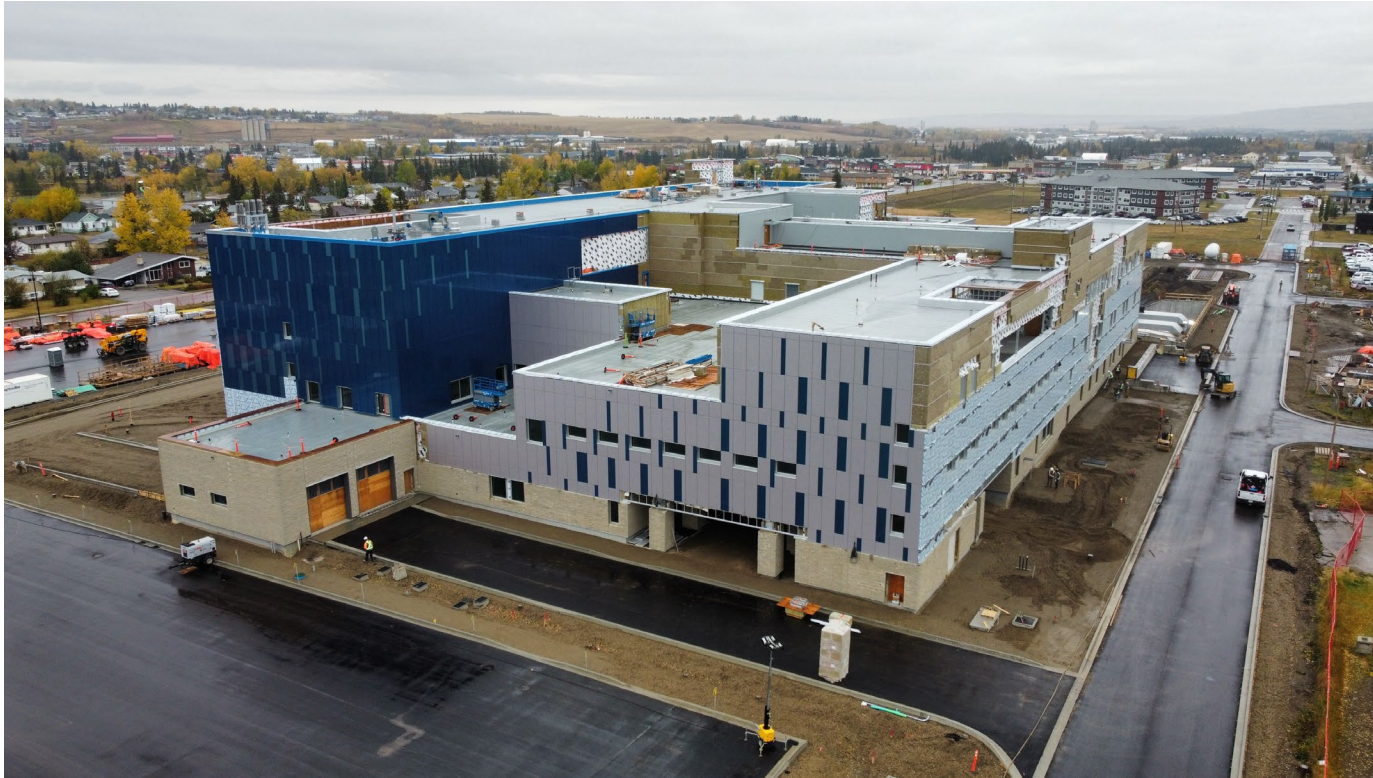
Ambulance Bays and East Wall of the Exterior
