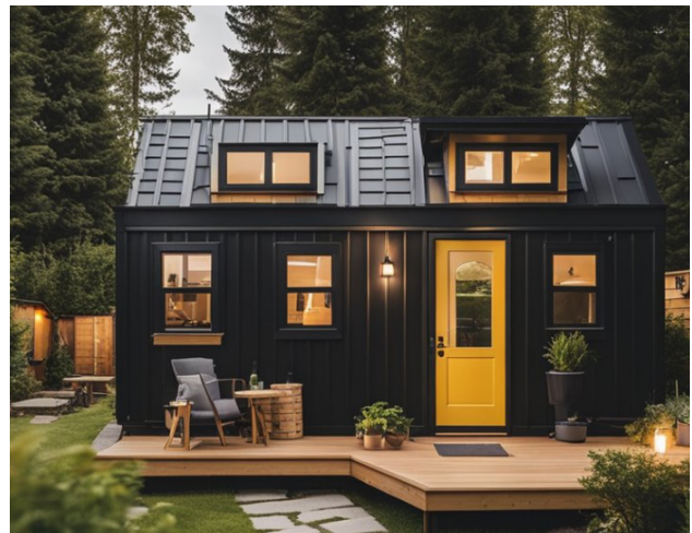
A tiny home which functions as a building must meet BCBC requirements.
